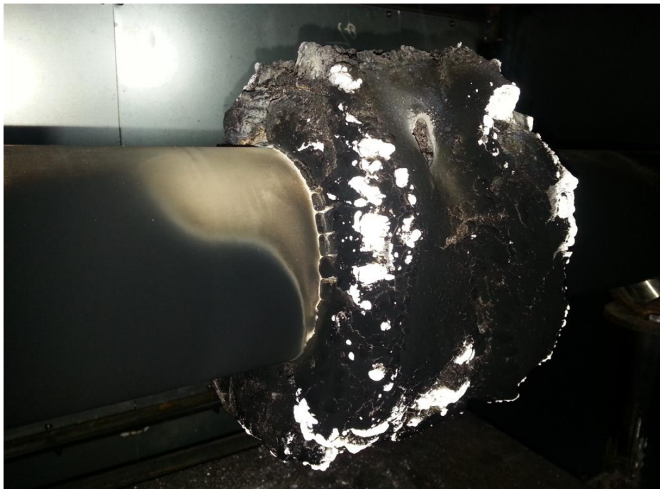
Photo 5-6. No leakage or visible cracks
