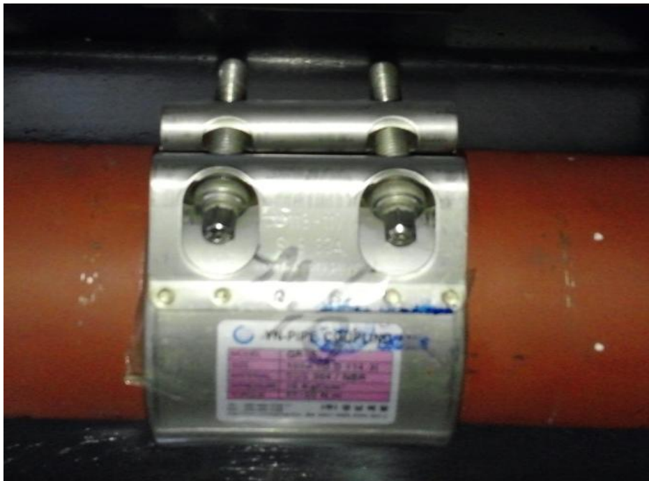
Photo 2-3. No sign of leakage or damage
