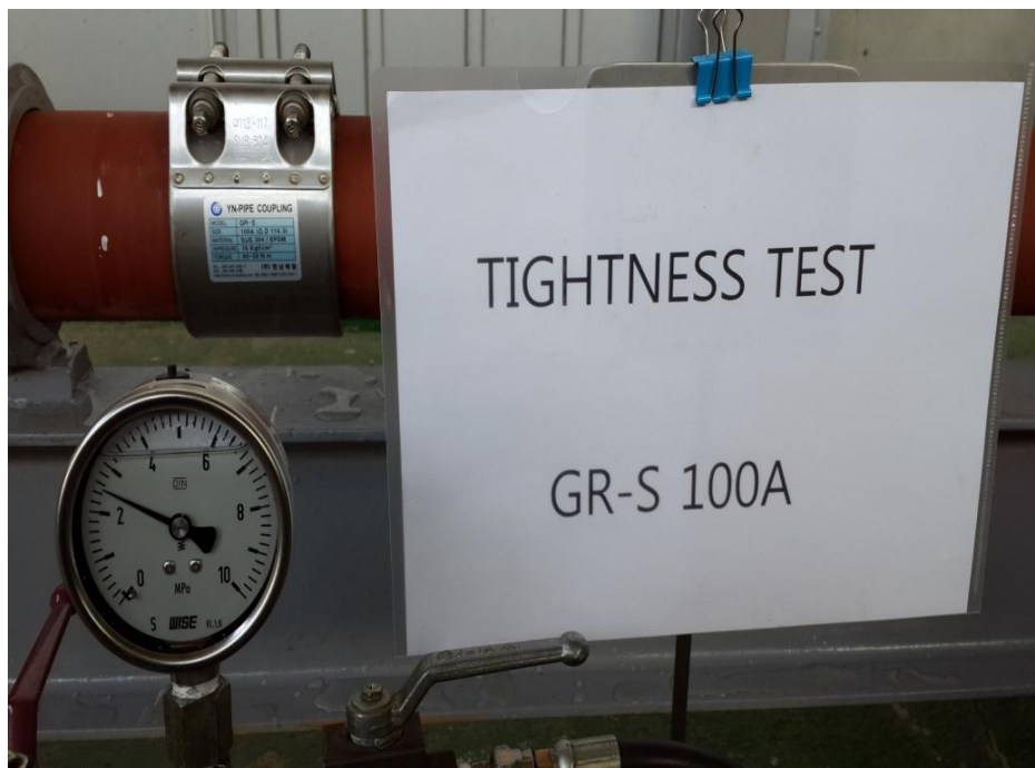
Photo 1-2. Test Pressure of Tightness Test
